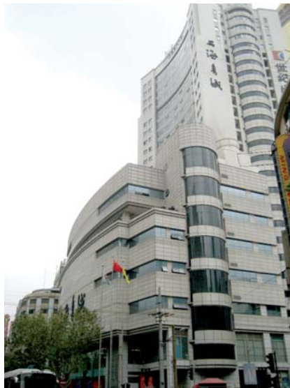
The building that houses the Shanghai Book City where books are sold on the first five to six floors.
